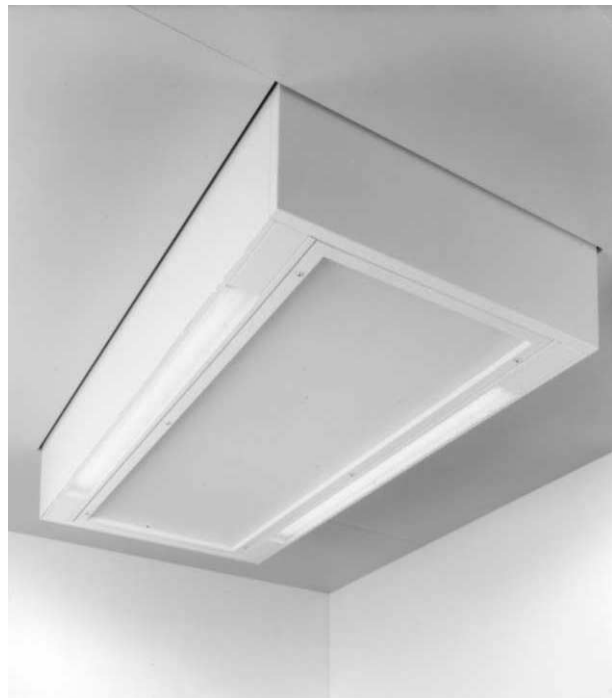
Dissection outlet installed in ceiling
