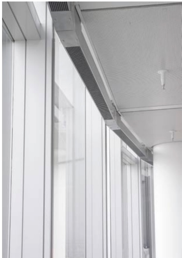
LUVAS profile system as rail at ceiling height
