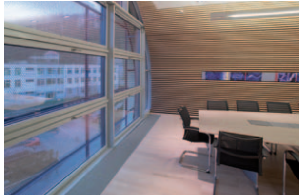
Fig. 1: Rectangular floor displacement outlet in front of a facade
