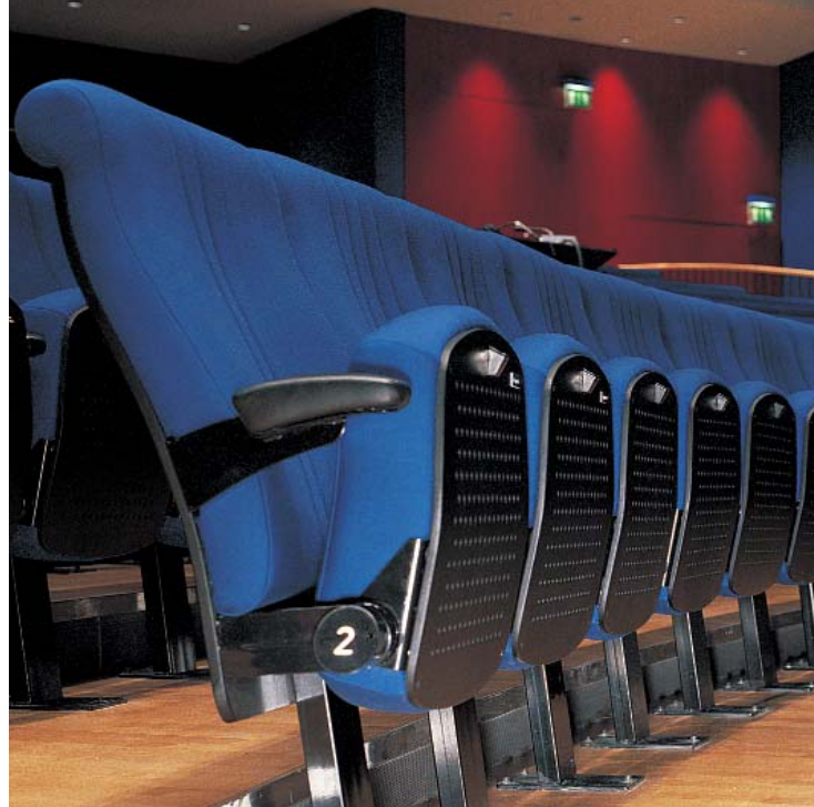
Step displacement outlet, type Q-SL, at Theater Hof, Hof/Saale / D
