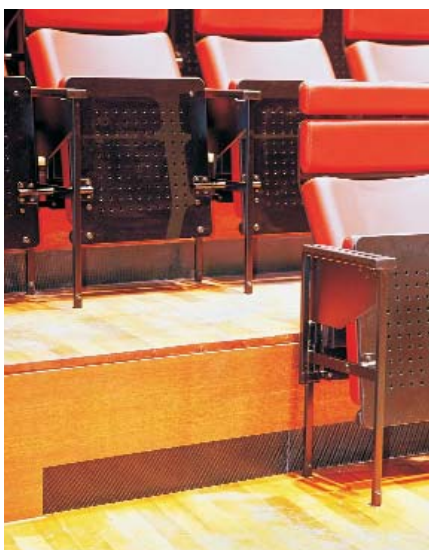
Step displacement outlet, type Q-SL, in the auditorium of the Nordic Embassies, Berlin / D
