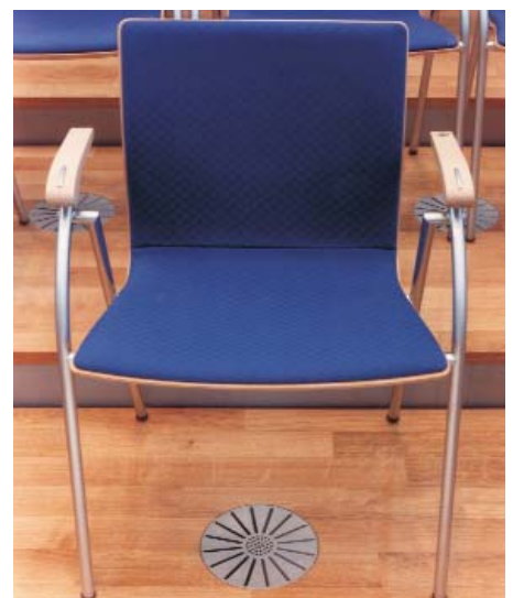
Figures above: Floor displacement outlet, type Q-B-DN 200, at 'Congress Center Messe Frankfurt', Frankfurt am Main / D
