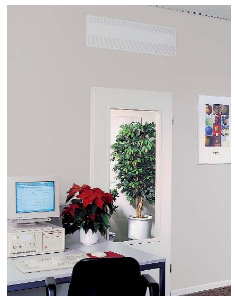
Wall displacement outlet, type Q-WK, in an office
