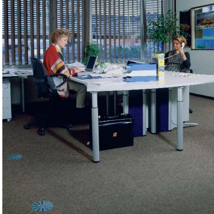
DN 150 in an office
