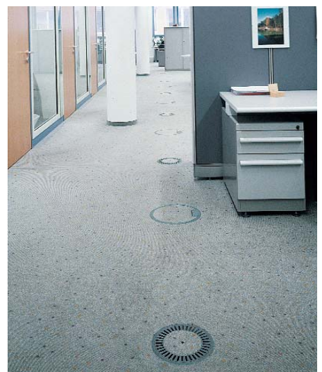
NTK floor twist outlet in an open-plan office of Carl Schenk AG, Darmstadt / D
